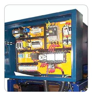
The SCM controls flow of oil to the rig from the ring main. It is controlled by the PULSAR software in off/low/high pressure mode, with a safety pressure switch to shut the rig down if sudden unexpected pressure changes are detected. From here, the oil is distributed to the individual servovalve manifolds through flexible hoses.
